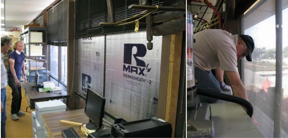
Left: Rob Braun (left) and Steve Hughes install insulation sheets in west-facing window frame. Right: Bob Palazzola vacuums behind filing cabinets before installation of foam insulation.
